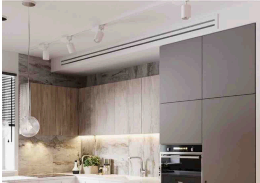
rails and spots are attached to the ceiling
